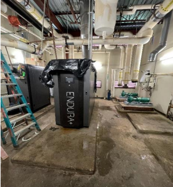
New Boiler Installation at Parkwood Hill IS
