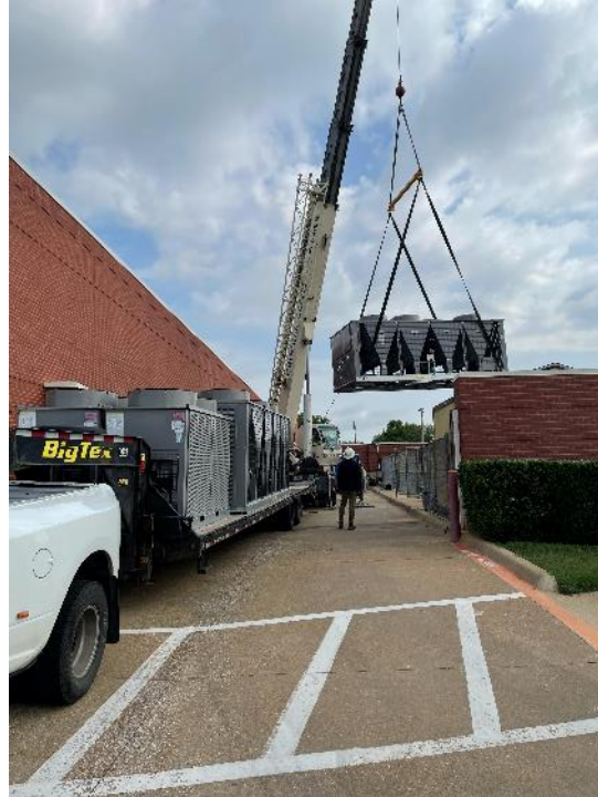
New Chiller Installation at Park Glen ES
